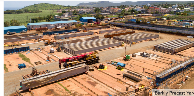
Barkly Precast Yard
