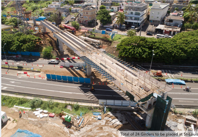
Total of 24 Girders to be placed at St-Louis
